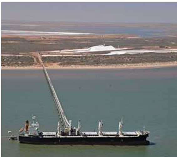
Figure 2 Photograph showing the Onslow Salt Jetty with ship alongside (Source: www.salt.com.au )
